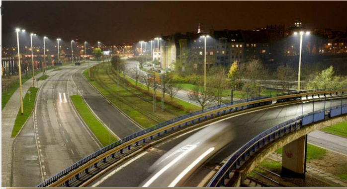
Public Street Lighting with Energy Saving Lamps
